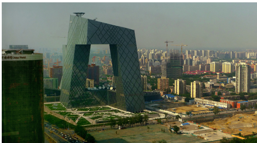
Fig. 1 China Central Television (CCTV) Headquarters, Beijing, OMA
