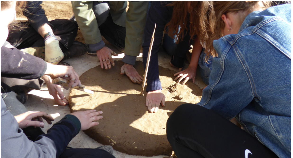
Top: The materials are stamped together Bottom: Defining the bottom of the tandoori oven
