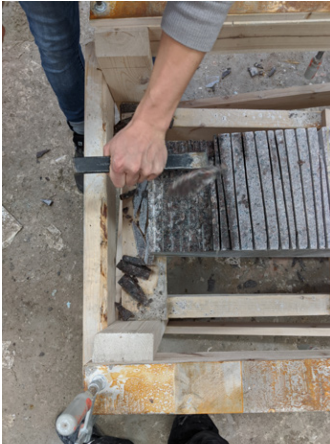
The large granite blocks for the pile foundations come from a quarry on the Danish island of Bornholm. With inspiration from traditional Japanese construction techniques, the tops of the blocks were cut to form an overlapping joint with the piles.
