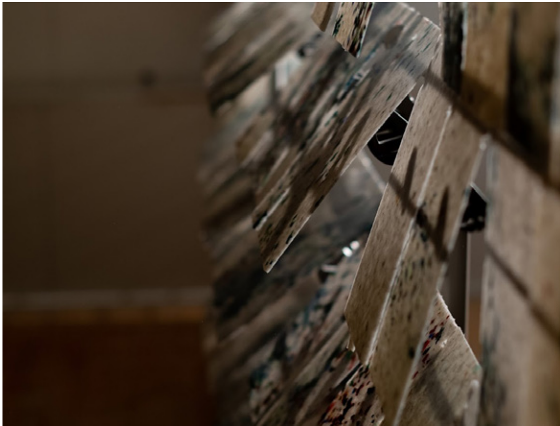
Detail of the shingle cladding wall showing mechanically controlled cranks that open selected shingles
