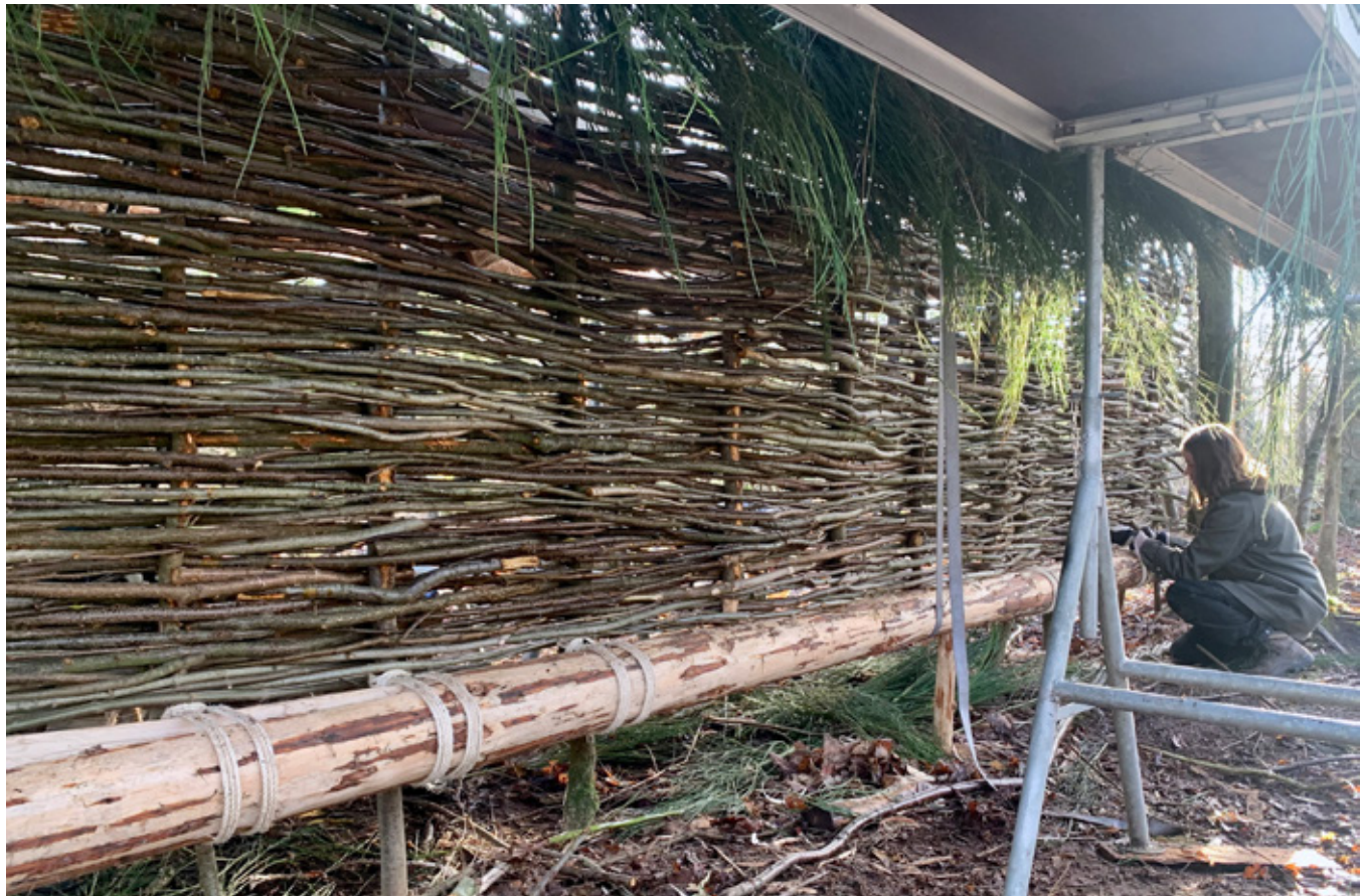
Screen for a cattle shelter made from vertical stakes interwoven with horizontal withies, a technique known from older timber frame construction. The material is black cherry, Prunus serotina . The Danish Environmental Protection Agency designates this as an invasive species that should be destroyed, and as it is present in abundance it represents a free resource. The wood is hard and strong but also pliable, almost like bird cherry.
