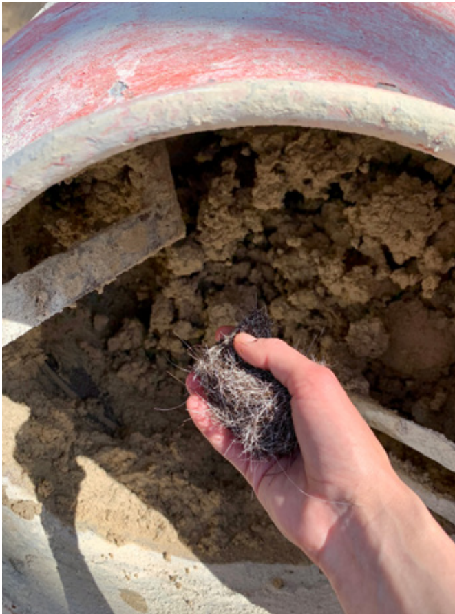
Lime mortar from a nearby mortar mill is used in the construction of the cobblestone wall. The mortar is reinforced with hair from the horses at the Hjerl Hede open-air museum.
