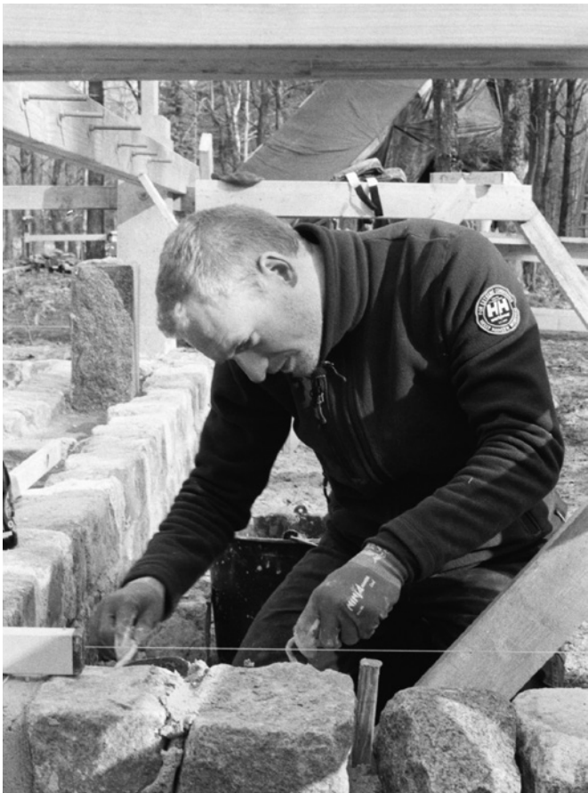
With each course in the core-and-veneer wall, clay is rammed into the core to stabilise the cobblestone walls. In addition to keeping the animals and the deep litter in, this technique also helps stabilise the granite pile foundations.
