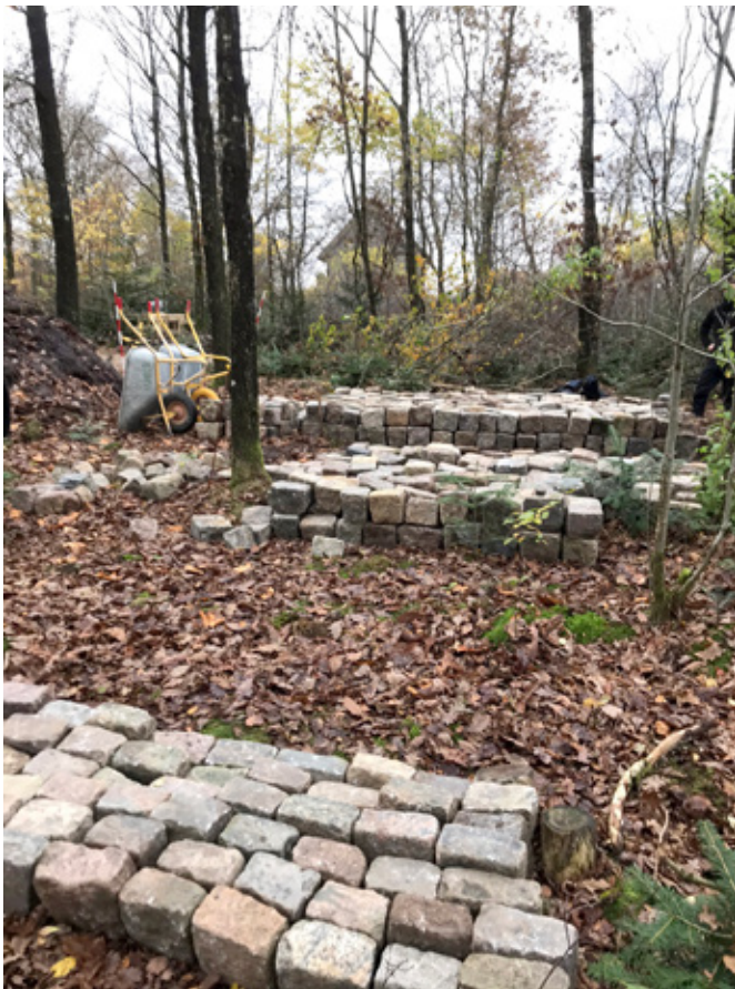
Cobblestones sorted by size and ready for building. The stones were previously used in the driveway to the open-air museum Hjerl Hede; before that, they paved the main street in the Danish town of Skive.
