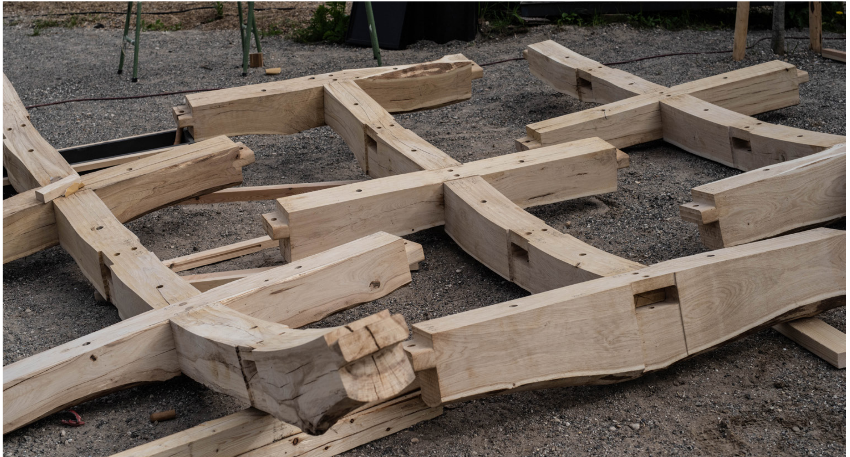
In the construction of the prototype, the beams were first assembled in rows and then pulled together with clamps. Next, the assembled construction was lifted into place in the frame by crane.
