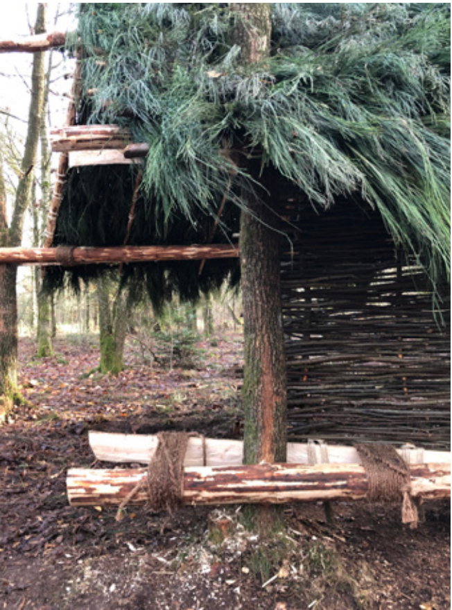
The cattle shelter is built entirely from organic materials, meaning that the construction will be composted and dissolve into the forest floor if it is not maintained. The roof is suspended from the trees that also support the walls, so that the building literally has no 'footprint'. The flexibility of the lashed joints allows the living trees to grow and to move in the wind.
