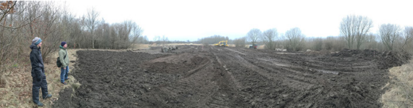
The recipient area in Eskelunden is being prepared, February 2017. The nutrient-rich topsoil was removed to make room for the transplanted urban natural habitat from the goods railway site.
