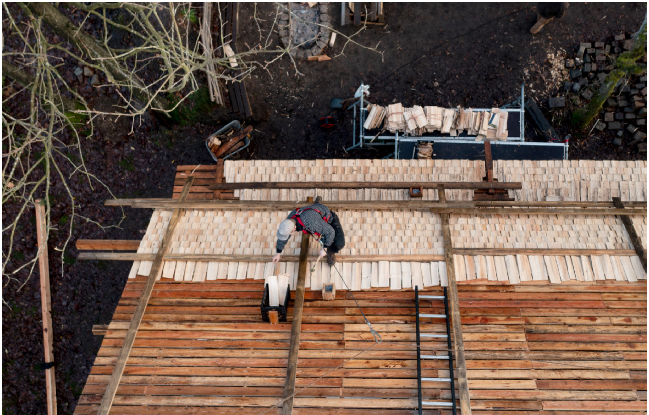
Roofing using shingles made from local common spruce.
