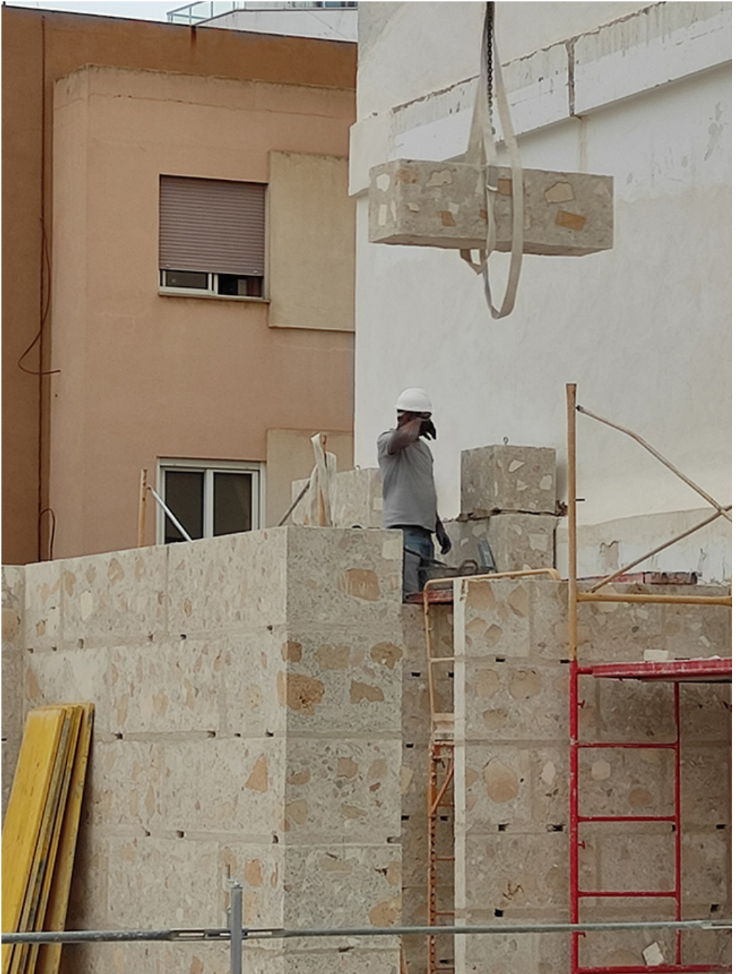
Demolished Marés stone, reused in IBAVI housing by Harquitectes, Palma
